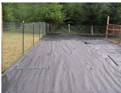
Here's a photo of the fabric installed in Kent's barn paddock. Kent tells us, “At minimum, my overlaps were two feet, but in most places I made them about four feet to allow for shift as the gravel is added and spread about. You can also see that I laid t-posts across the fabric for added support until we top it with 5/8" minus because of our evening coastal westerly breezes.”
