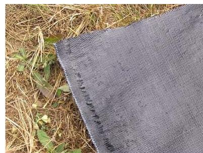
After this photo was taken, Kent also tucked the fabric under the fence and staked it on the outside. This will prevent horses from pulling the fabric up along the edges or by the gates.
