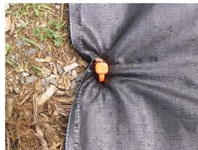
This is a 12" plastic tent stake that Kent used to hold the areas where seams met and high traffic places such as near gates. Kent notes that, “tent stakes work really well, but one needs to be careful not to hammer them completely through the fabric itself.”
