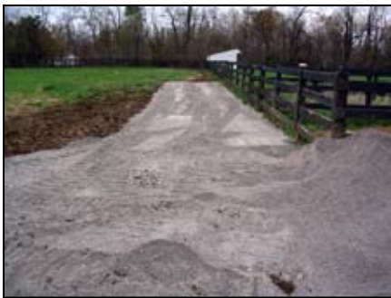
Figure 7. Surface layer of crushed stone.
