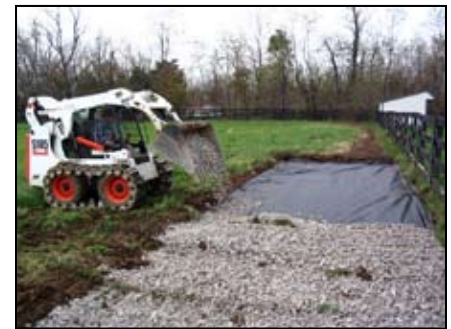
Figure 5. Base layer of crushed stone.
