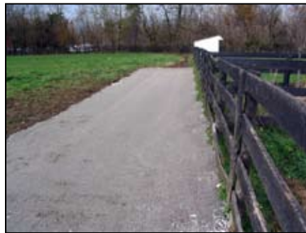
Figure 10. Compacted surface layer.
