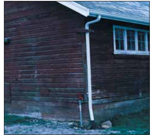
Gutters and downspouts reduce mud by directing water away from high-use areas.
